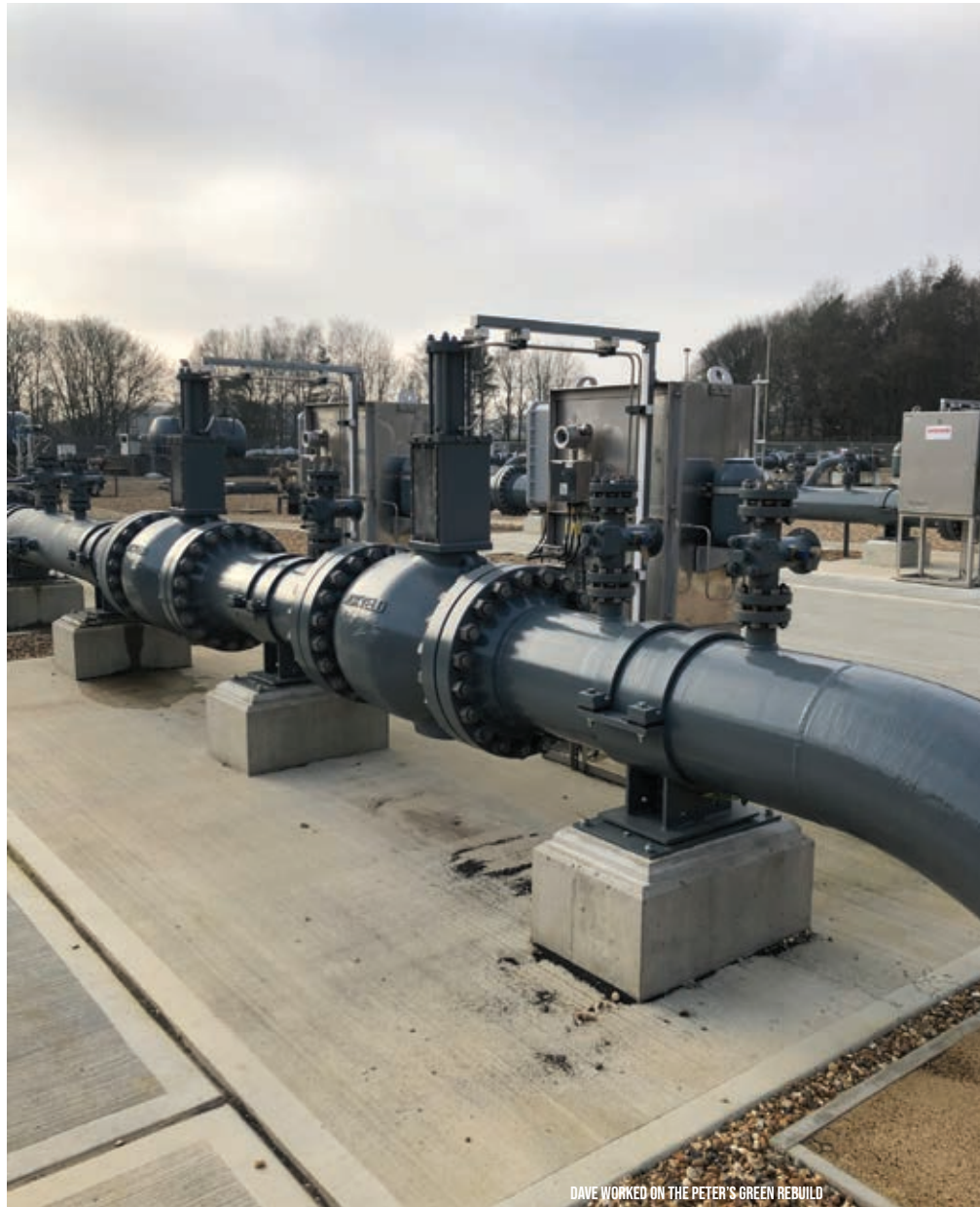
DAVE WORKED ON THE PETER'S GREEN REBUILD
