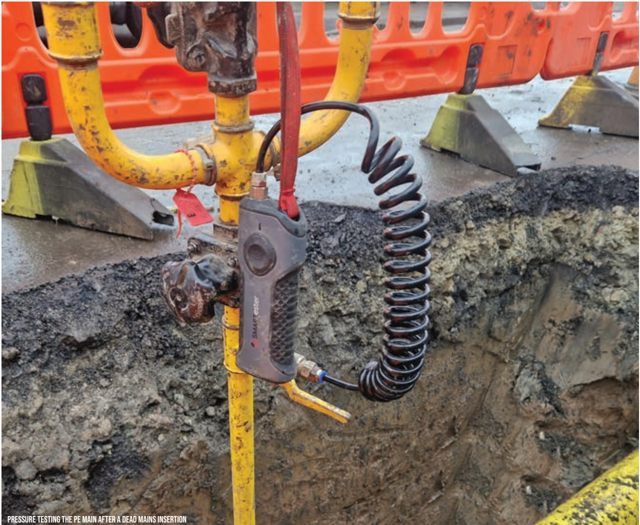
PRESSURE TESTING THE PE MAIN AFTER A DEAD MAINS INSERTION
