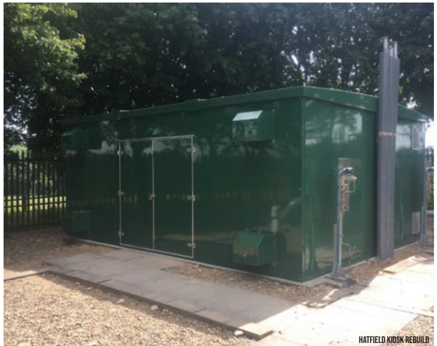
HATFIELD KIOSK REBUILD
