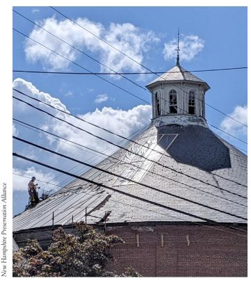
Yankee Steeplejack Co. crew repairing slate roof of the Concord Gasholder.
