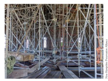
New steel shoring towers supporting compromised roof of the Concord Gasholder.
